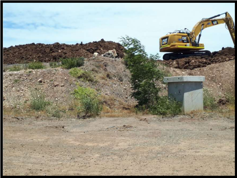
Figure 5: Site inspection photo dated 5 December 2019
